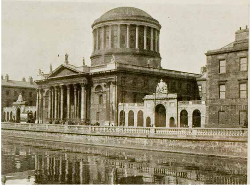
The Four Courts. (Dublin and the "Sinn Féin" Rising, Wilson Hartnell & Co., 1916).
